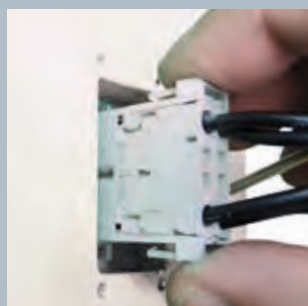
Snap in module insert from inside
